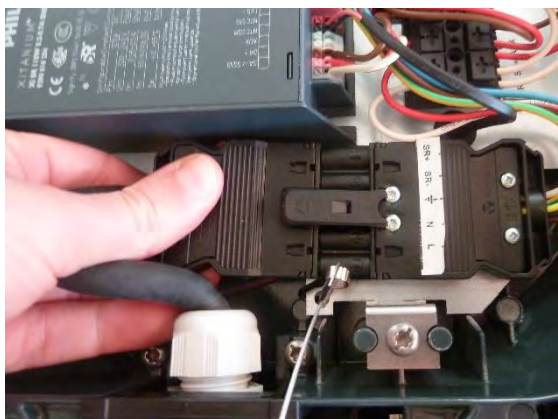
C - Disconnect the black power connector from the gear tray.
